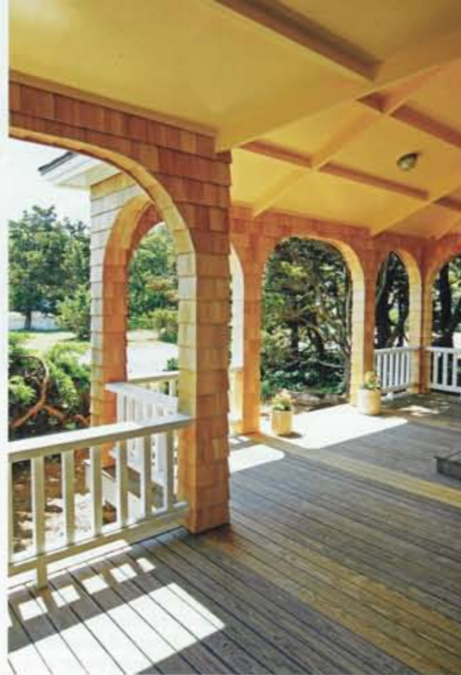
The porch restoration required 150 feet of custom railings, while the simulated camp style roof is actually a double roof for structural integrity.
